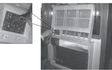
D Attach the front grille to the case by inserting the tabs on the grille into the slots on the front top of the case. Push the grille in.
