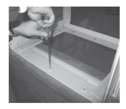
G Pull the accordion panels to each window sash track. Attach them on each side to the window sash and the window sill using 4 Type C screws.
